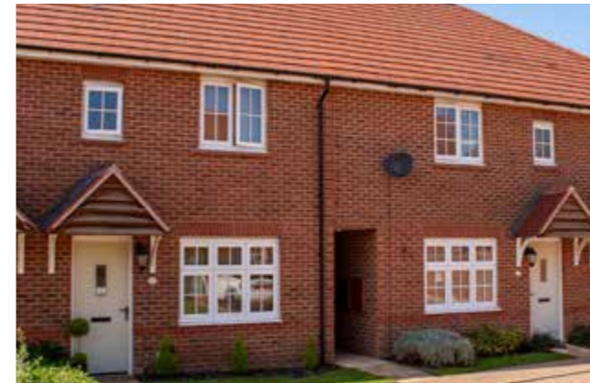
Providing ginnels in a terraced row is a traditional alternative to long narrow passageways around the rear of plots
