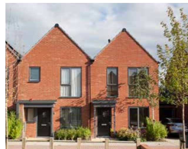
Gable frontages and varied fenestration add interest
