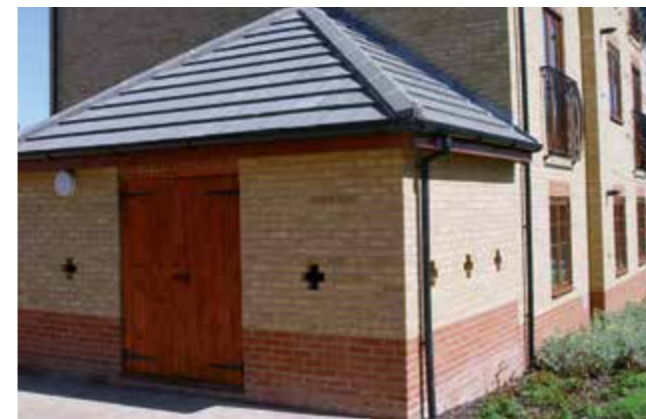
Example of a communal bin store serving apartments
