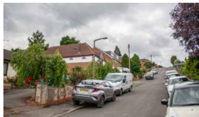
Residential development on a steep slope at Standhill Avenue
